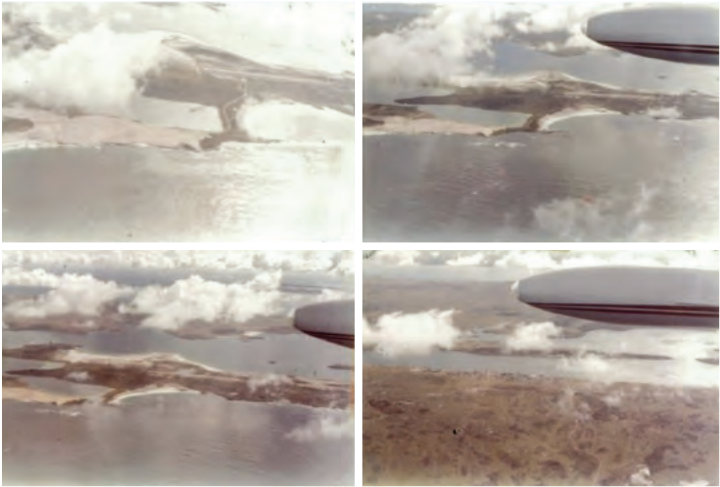
View of BAM Malvinas runway after the TC-23 survey on 18 April - Photo courtesy of: 1 st Air Photographic Group Archives
